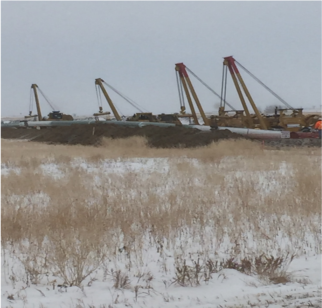
LOWERING PIPE INTO TRENCHES
