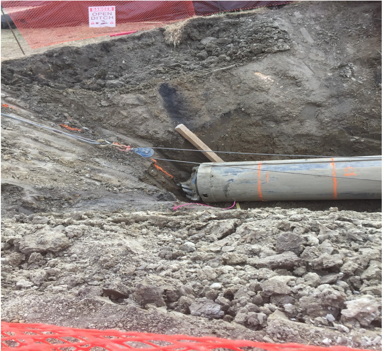
Bore drill bit for underneath roads.
