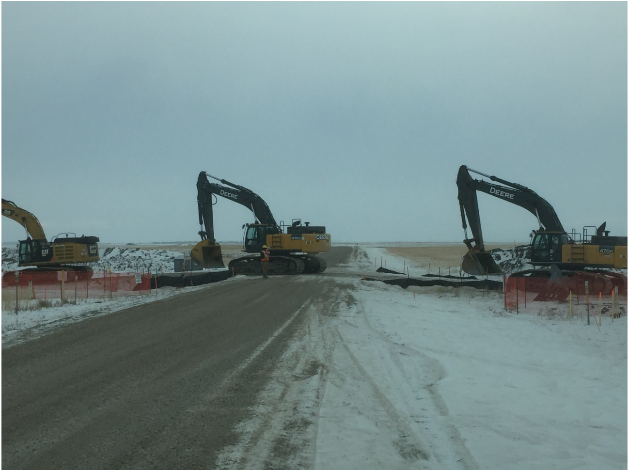
Excavators crossing roads
